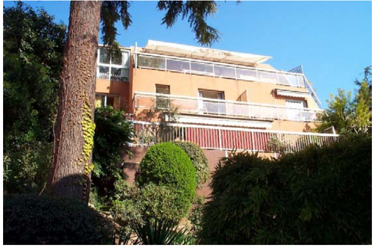
The apartments set into the hillside
